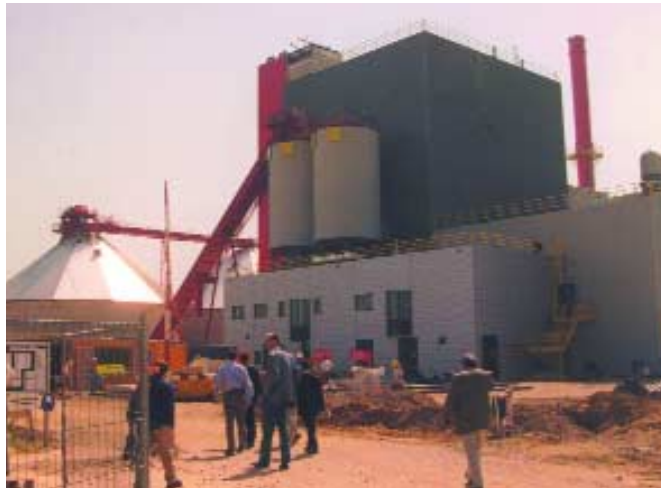
A 25 MW e woodchip fired power plant in Cuijk, The Netherlands with Bubbling Fluidised Bed (BFB) boiler.
