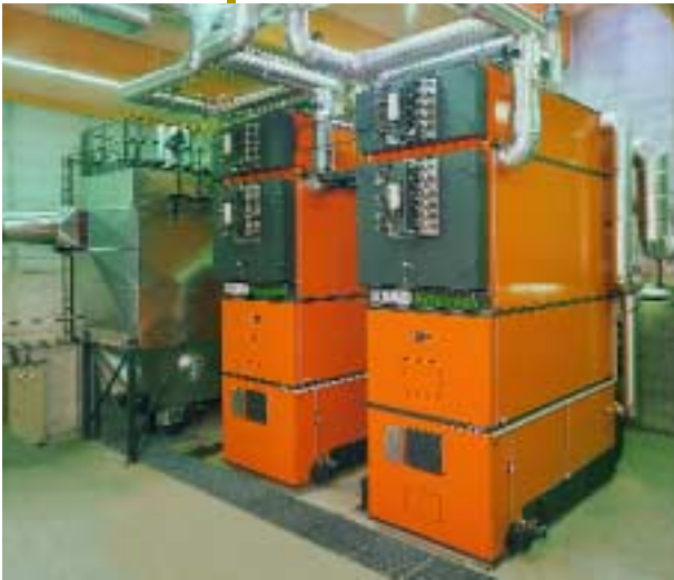
Two 3.2 MW th grate furnaces for wood chips, used for district heating in Interlaken, Switzerland. (Courtesy of Schmid AG, Switzerland)
