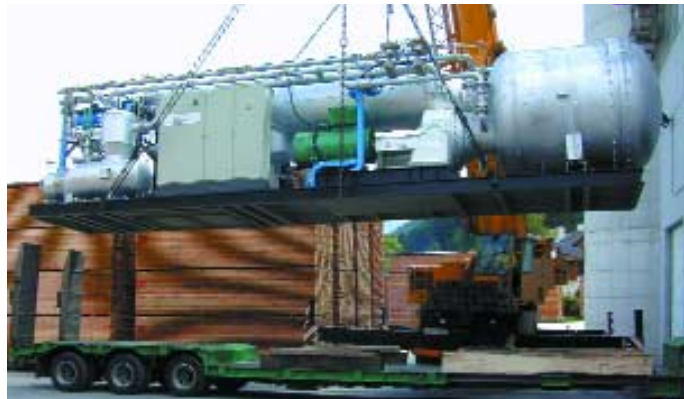
400 kW e ORC plant fired by a biomass grate furnace using sawdust and woodchips as fuel in Admont, Austria; the remaining heat is used for drying purposes and for district heating. (Courtesy of Turboden Srl, Italy)
