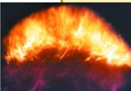
A view inside a step grate boiler. (Courtesy of TNO, The Netherlands)
